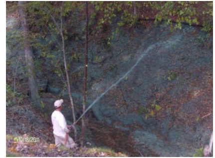
Ravine 3 - During Restoration
