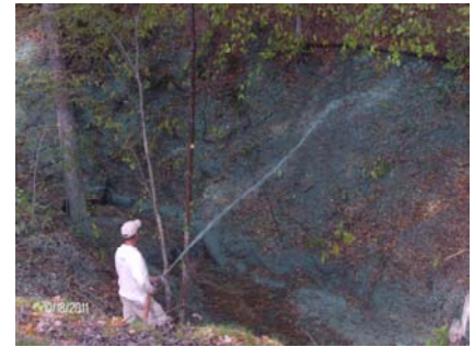
Ravine 3 - During Restoration
