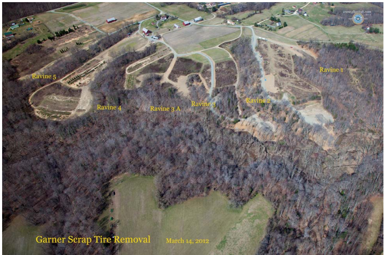
Aerial Photo of Entire Site During Cleanup
