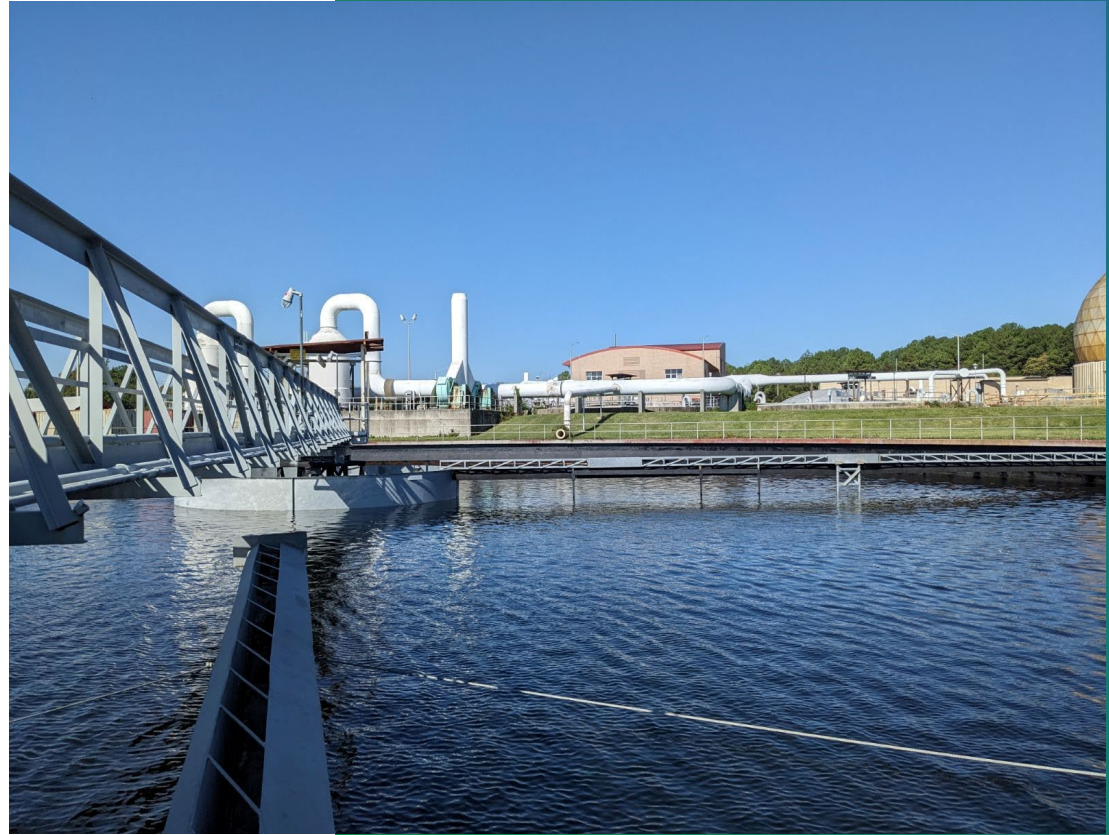
Primary Settling Tank
